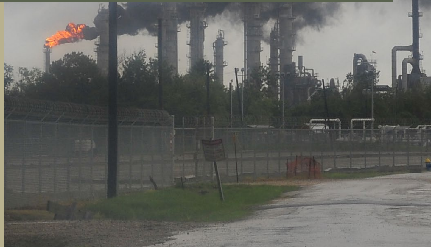
It Takes Roots. "Hurricane Harvey Disaster Damage." 2017. JPEG.
